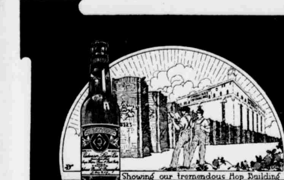
Showing our tremendous Hop Building
